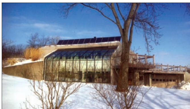
Fig. 6: Sidwell House, Raven Rocks, Ohio, USA / Malcolm Wells, 1990
