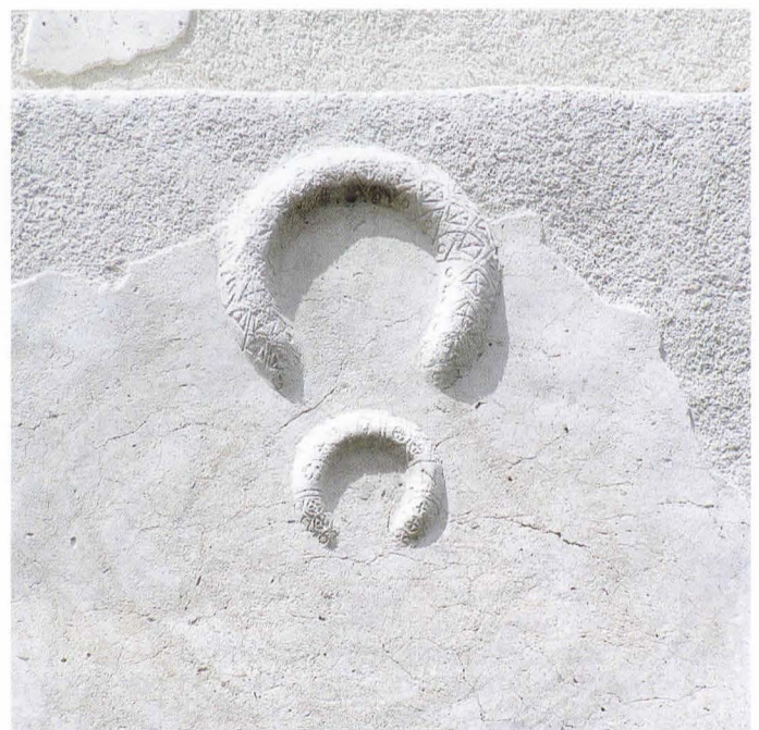
Fig. 30. Chancel apse. The same zone, after restoration
