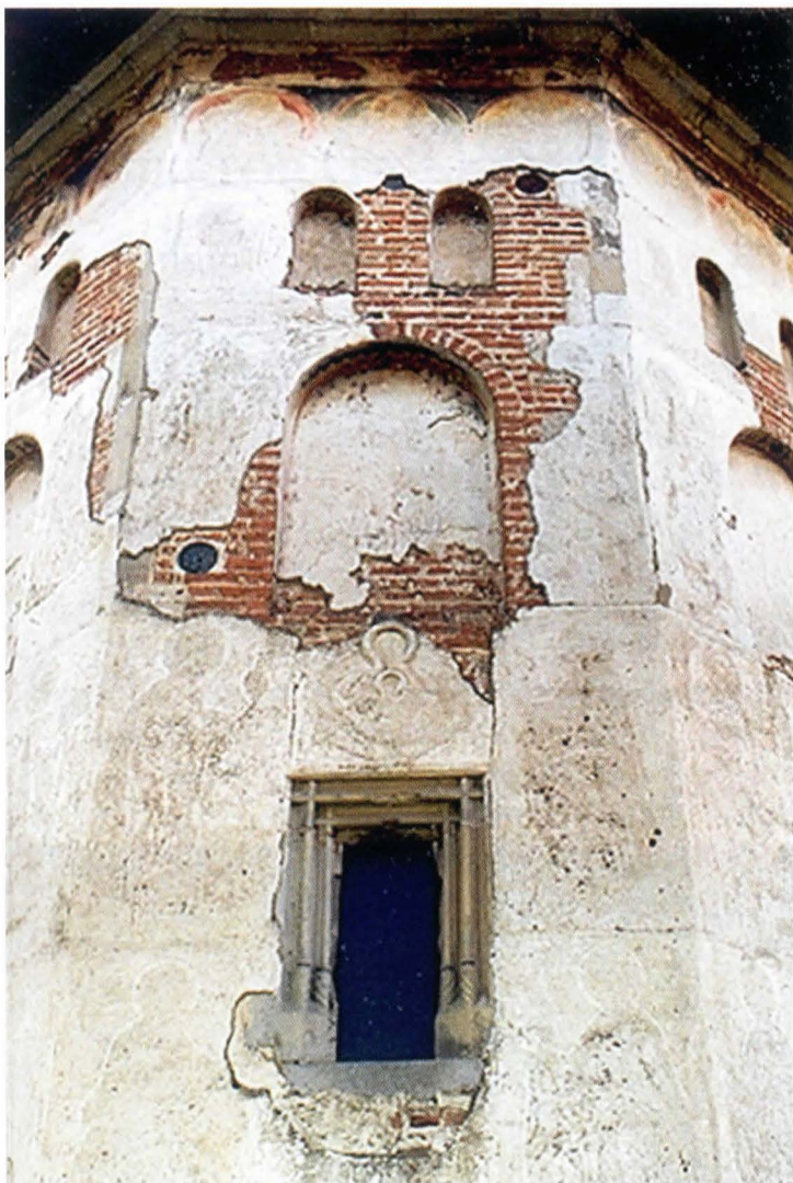
Fig. 27. Chancel apse. Before restoration
