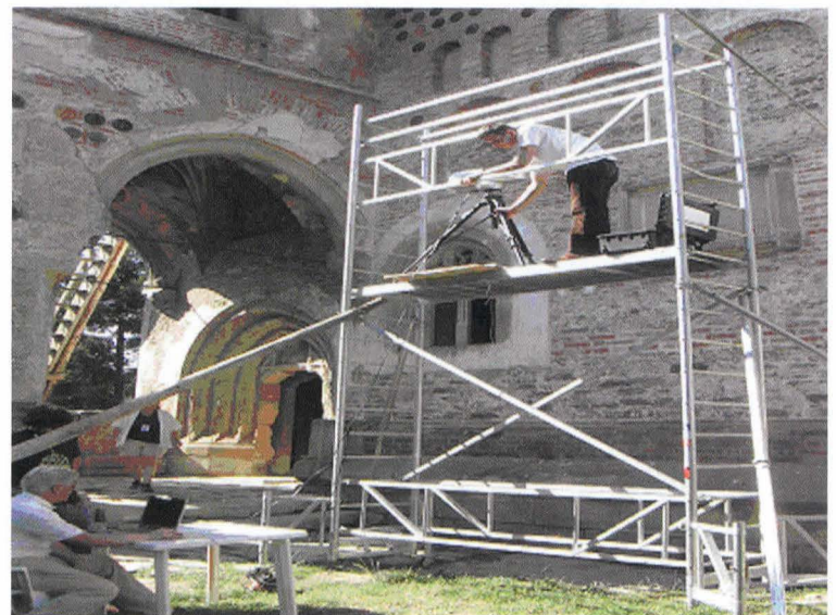
Fig 2.3 Scanner situated on a scaffold
