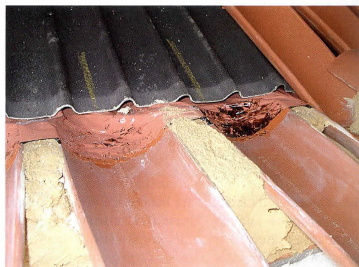
Fig. 13. Rain water protective element
