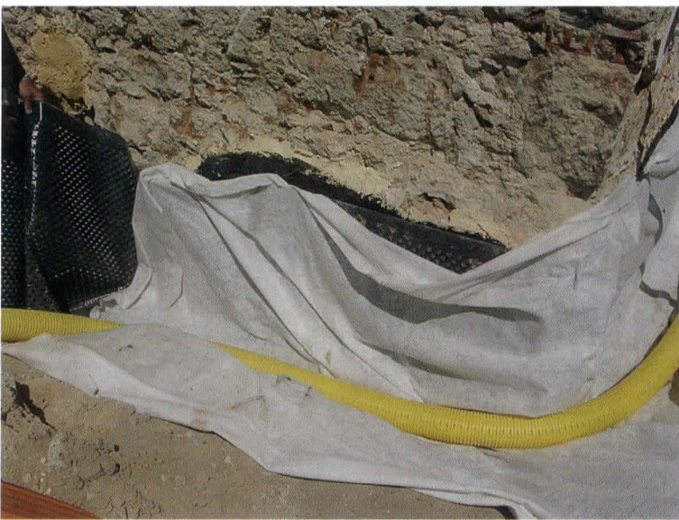
Fig. 6. Geo textil on draining solution
