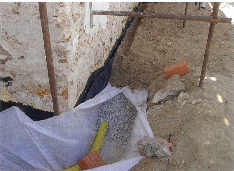
Fig. 7. Draining solution materials
