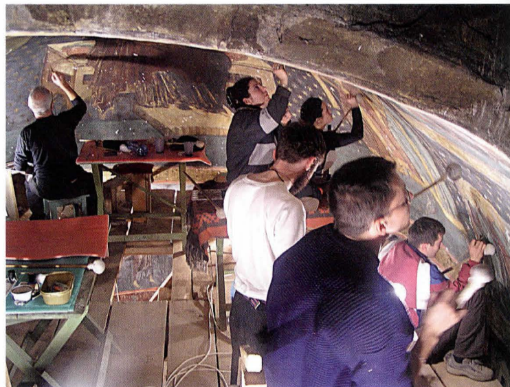
Fig. 26. During the restoration process
