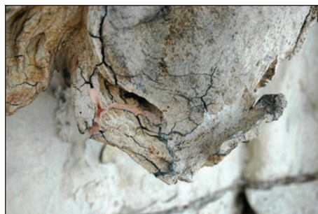
Fig. 19 - Colmatarea fisurilor prin injectare cu mortare fluide, fațada Lipscani / Clogging of the cracks by injecting fluid mortars, the Lipscani facade.
