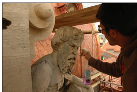
Fig. 19 - Colmatarea fisurilor prin injectare cu mortare fluide, fațada Lipscani / Clogging of the cracks by injecting fluid mortars, the Lipscani facade.
