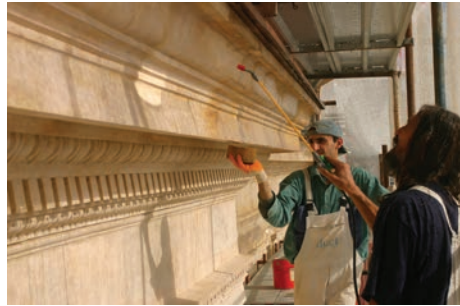
Fig. 24 - Tratamentele protective al suprafetelor de calcar cu o substanta hidrofuga, fațada Lipscani / Protective treatment of the limestone surfaces with a water repellent product, the Lipscani facade.
