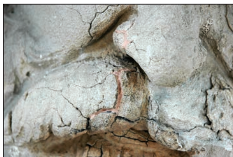
Fig. 19 - Colmatarea fisurilor prin injectare cu mortare fluide, fațada Lipscani / Clogging of the cracks by injecting fluid mortars, the Lipscani facade.
