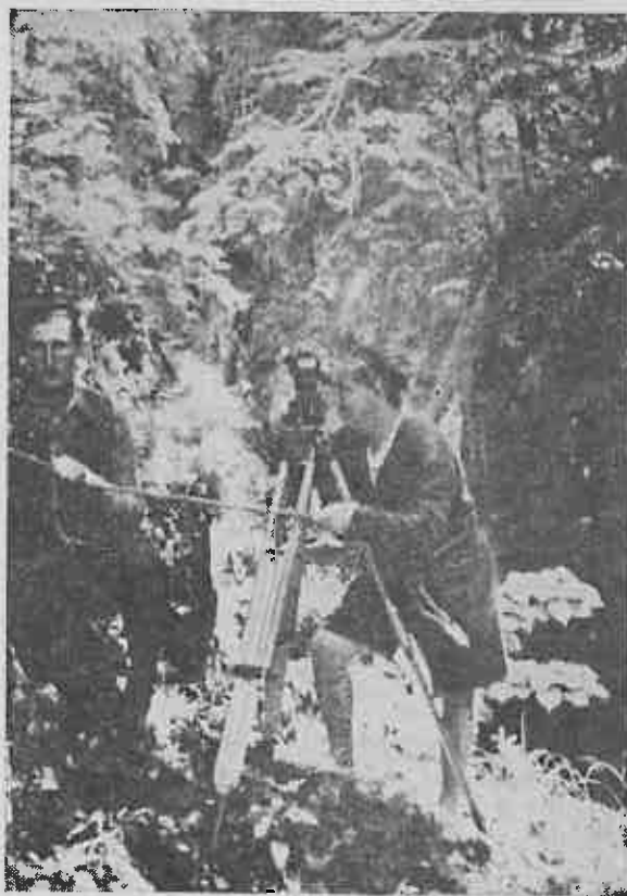
Fig. 6. Ridicînd profile transversale
