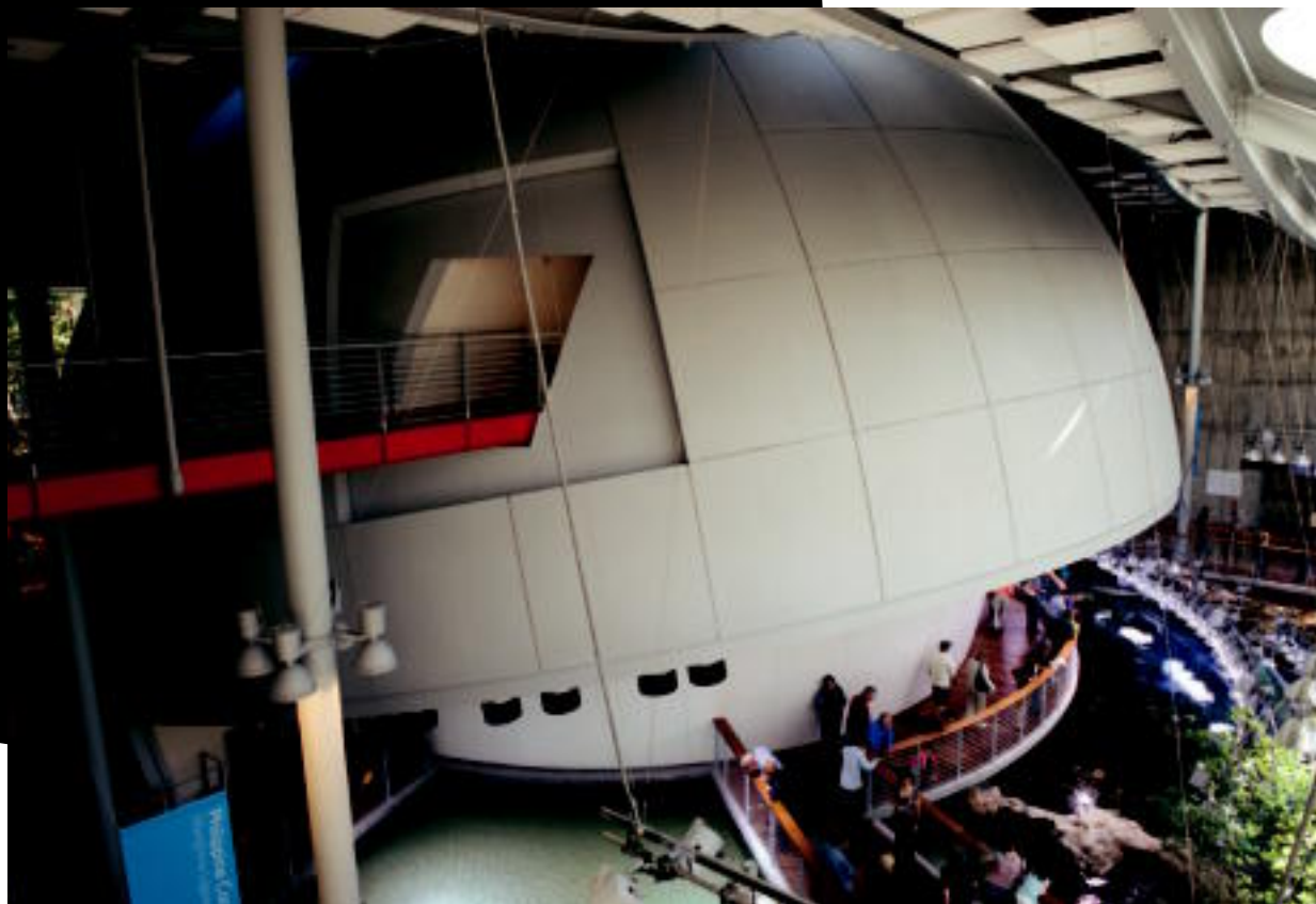
NO PLACE LIKE DOME The Morrison Planetarium's 90-foot-diameter dome is the most imposing structure inside the California Academy of Sciences. In keeping with the building's green design, the dome's structural frame is made of 100-percent recycled steel. Even when looking to the stars, the Academy is thinking about Earth.
